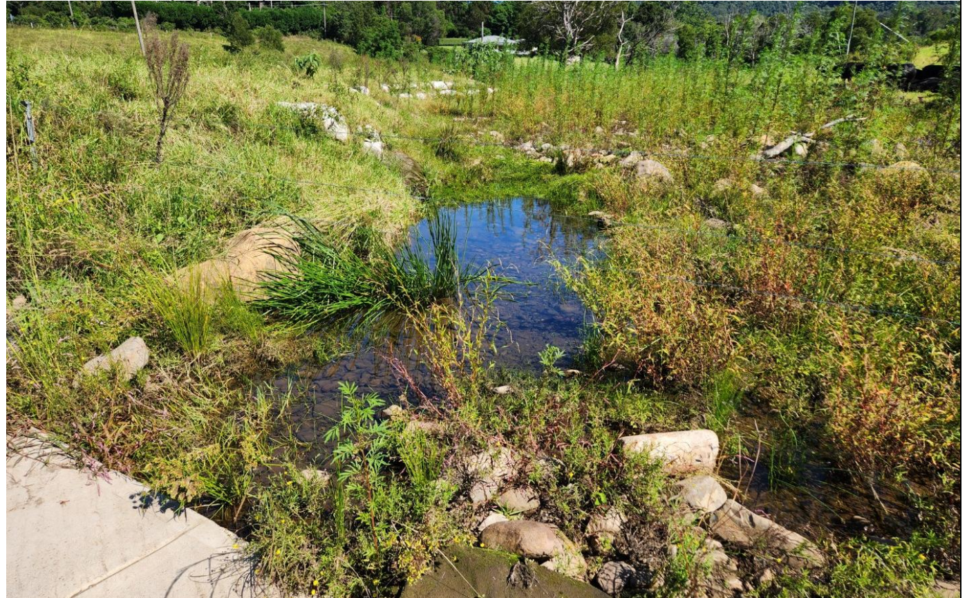
Photo 9. Site on 3 April 2025 showing erosion of south-west embankment, failed ELCO bags and accumulated rock (cf photo 7)
