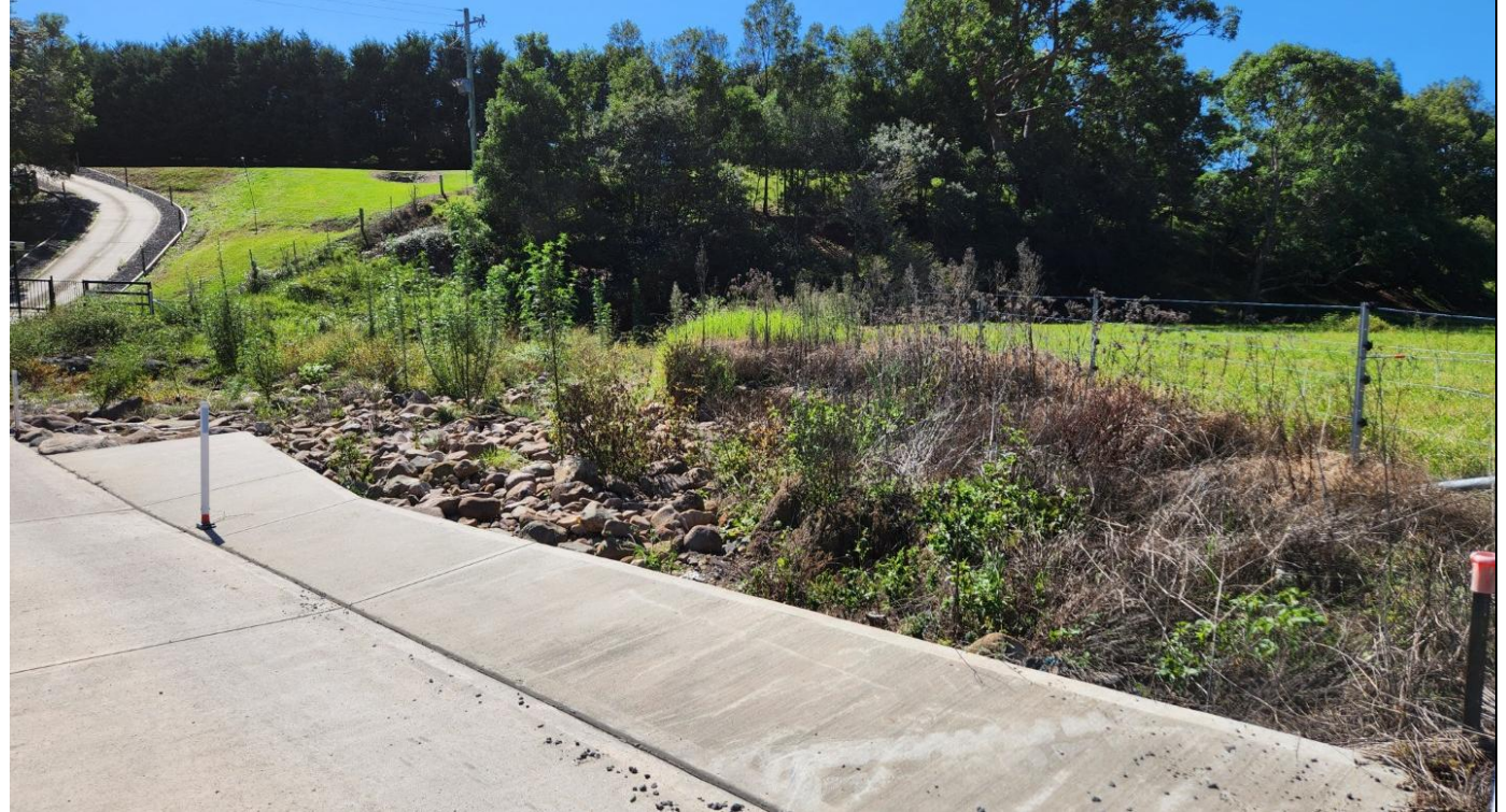
Photo 8. Site on 3 April 2025 showing erosion of south-east embankment and accumulated rock (cf photo 6)
