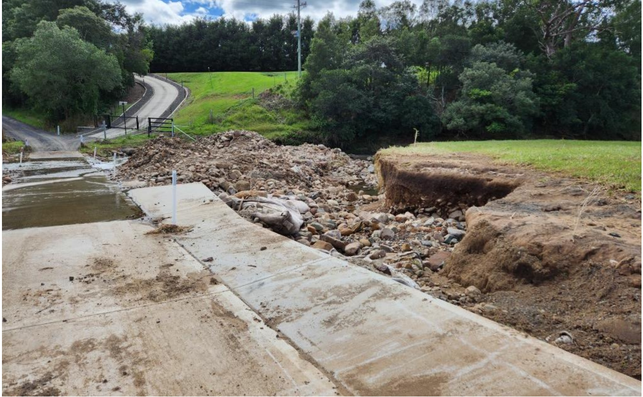
Photo 6. Post stabilisation works (11 April 2024) showing erosion of south-east embankment and accumulated rock
