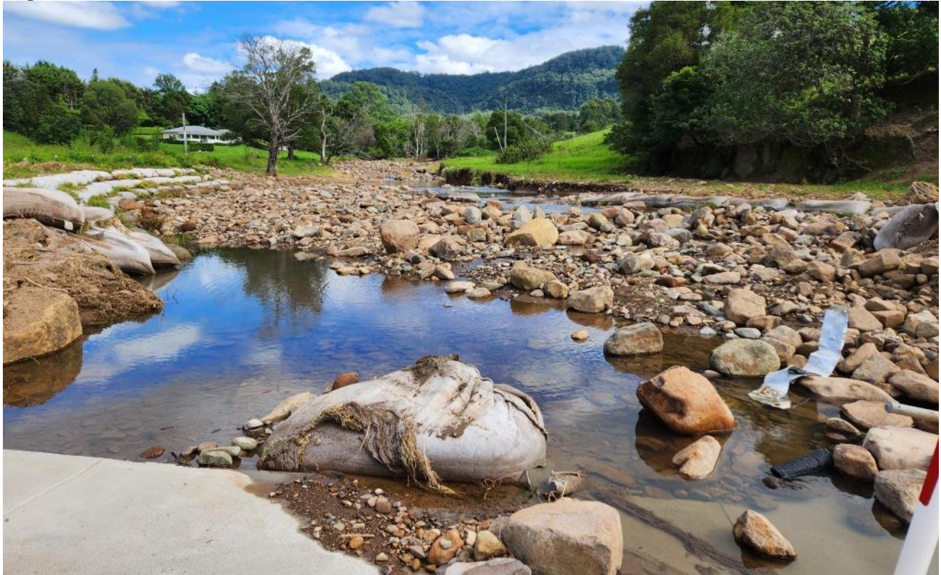
Photo 7. Post stabilisation works (11 April 2024) showing erosion of south-west embankment, failed ELCO bags and accumulated rock
